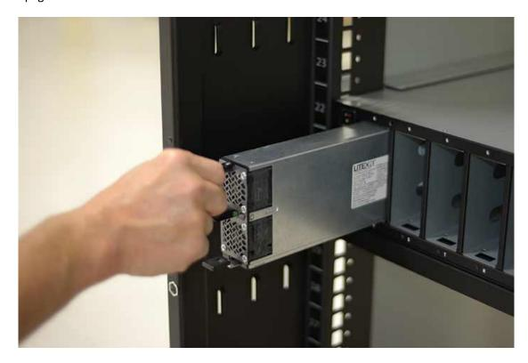
2. Slide the remaining PSUs into the empty slots in the Power Shelf until they click into place.
