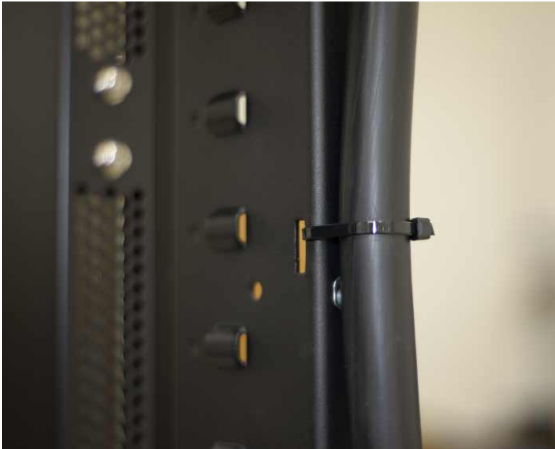
Power Cable secured to the Rack with Cable Tie
