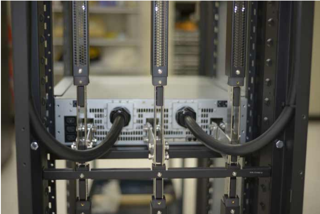
Power Cables routed along the Rear Vertical Support to the top of the rack inside Rack Extender Kit
