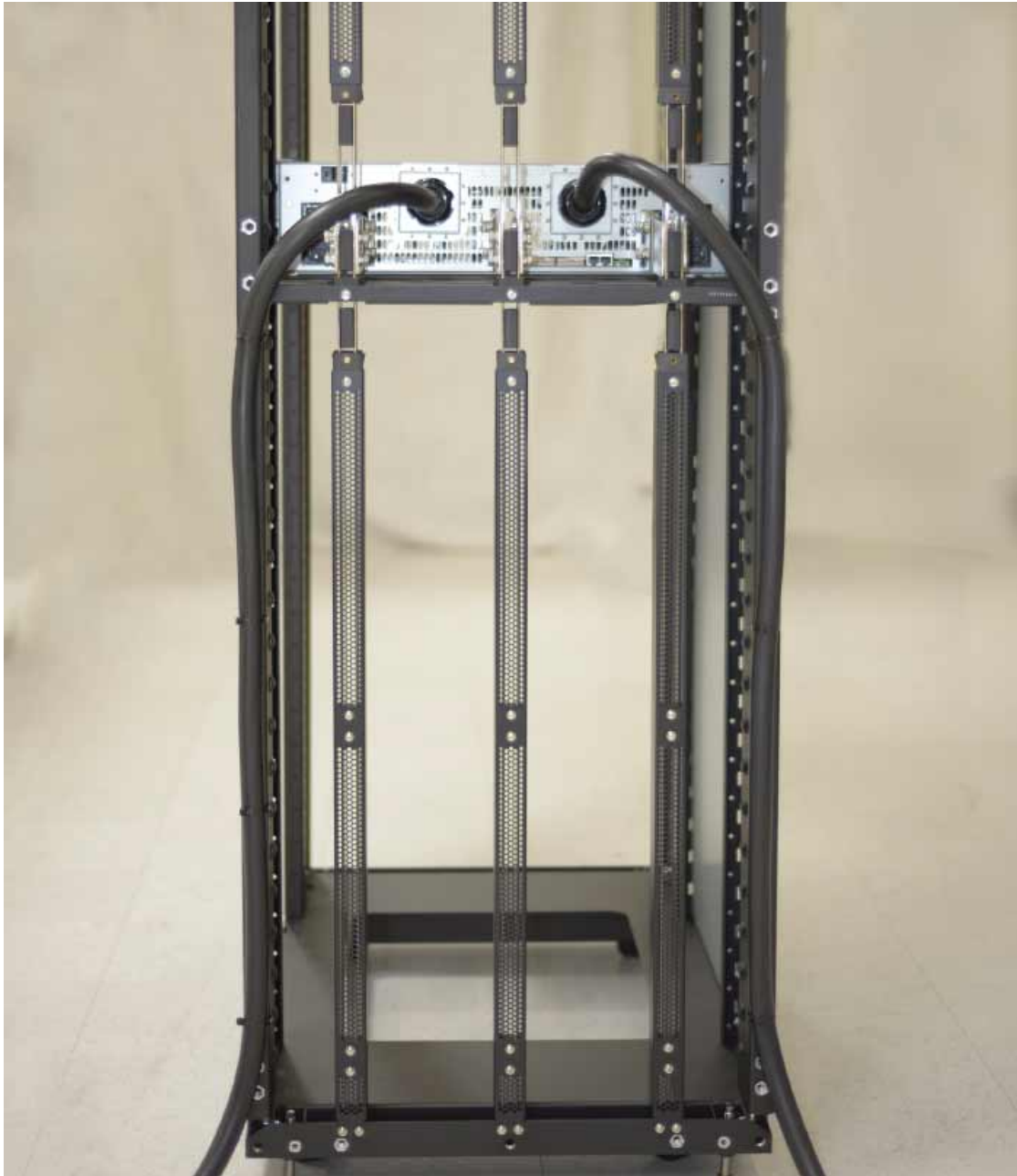
Power Cables routed to the bottom of the Rack
