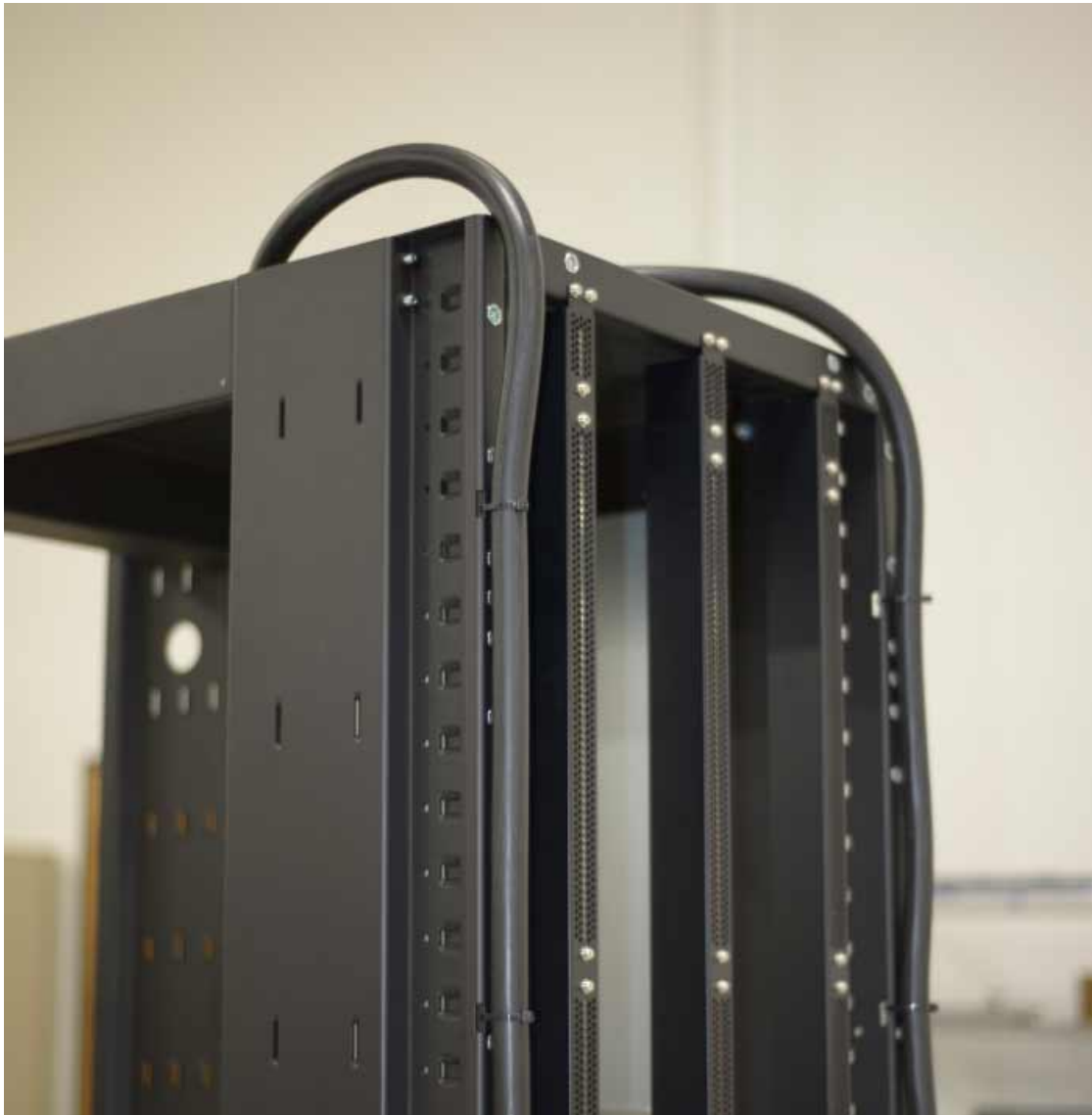
Power Cables routed to the top of the Rack
