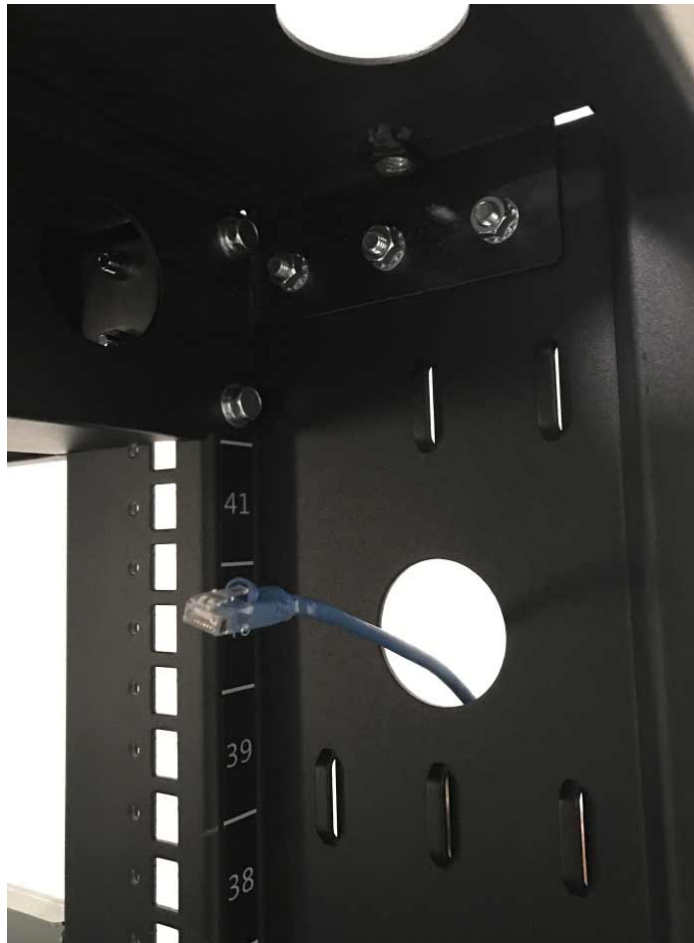
Signal cable routed through the side of the Rack
