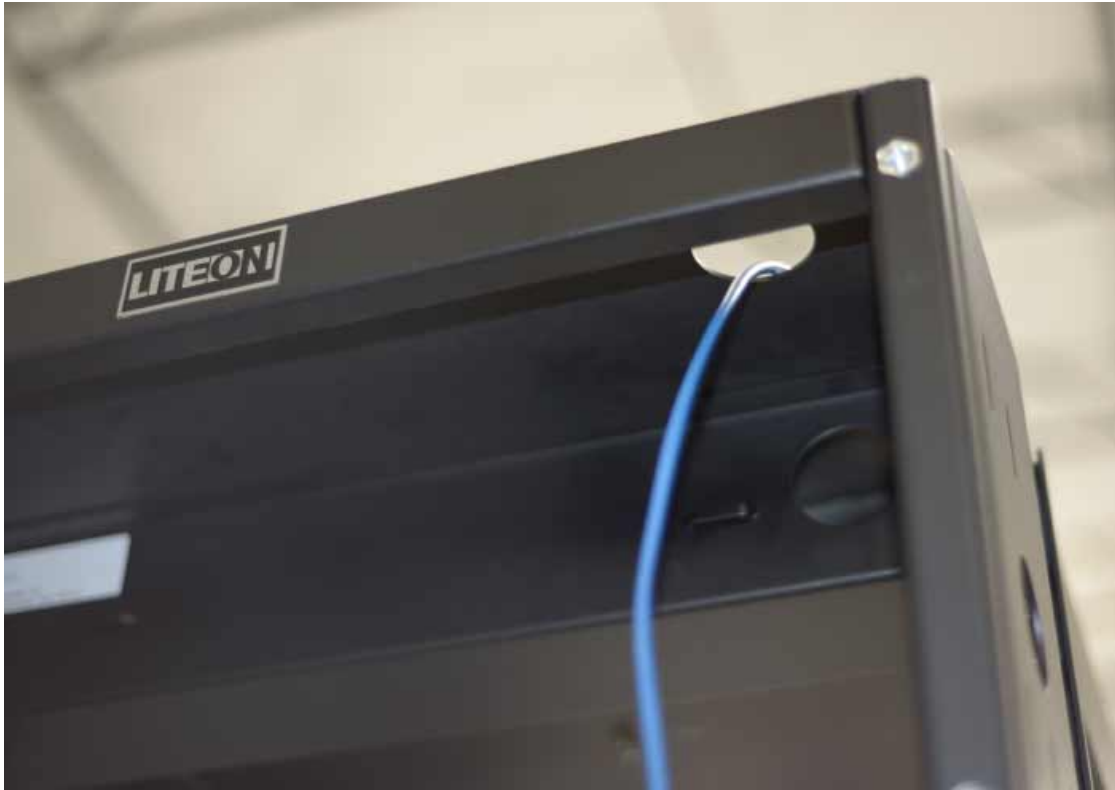
Signal cable routed through the top front opening of the Rack
