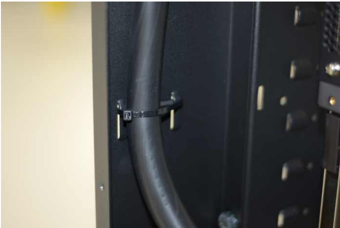
Power Cable secured to the Rack Extender Kit with Cable Tie
